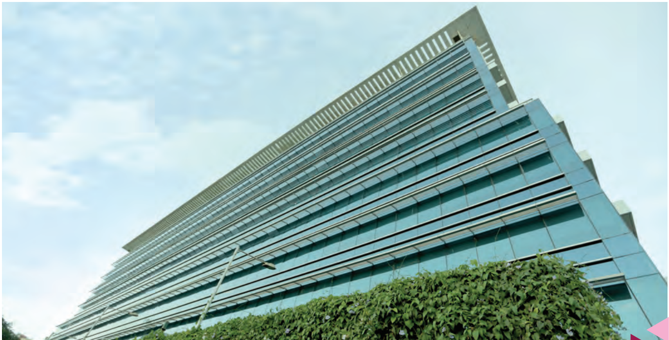
Axis House, Mumbai
