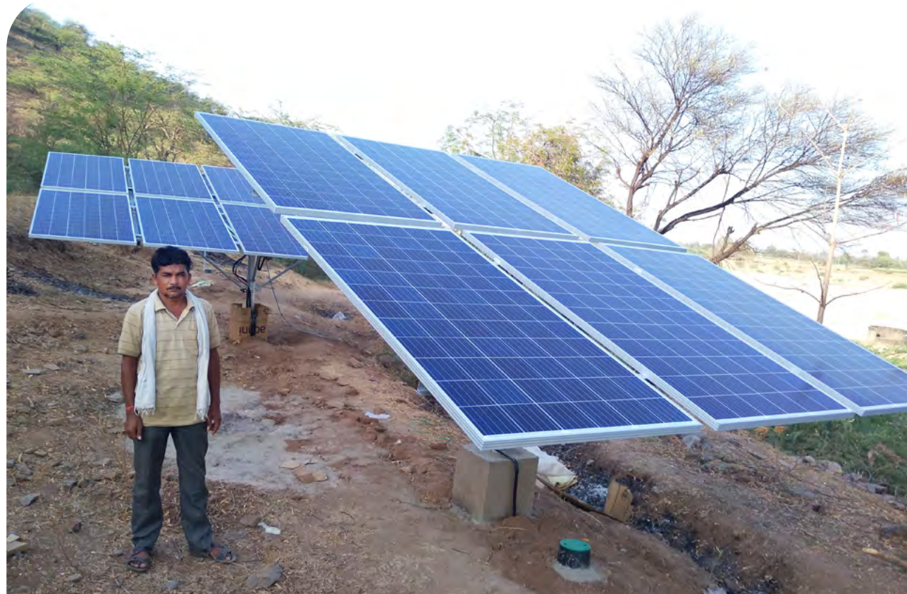
A Solar Lift Irrigation system in Banaskantha, Gujarat
