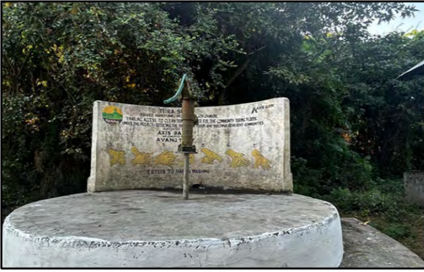
Figure 4: Raised Handpump
